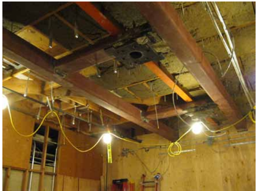
△ Wide-flange beams replaced wood frame load-bearing walls, allowing for larger operating rooms within the existing surgery suite space.
